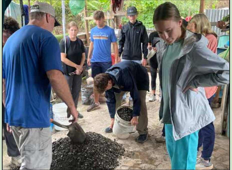
Concrete flooring project
